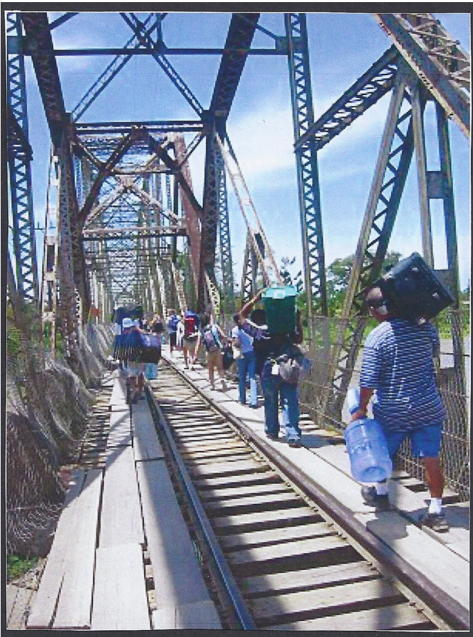
Fig. 13 – Bridge crossing the Sixaola River basin at the border near the Caribbean Sea.
